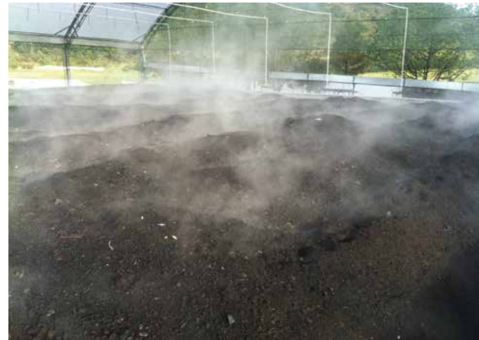
Test and demo plant with the COMPOnent aeration system
