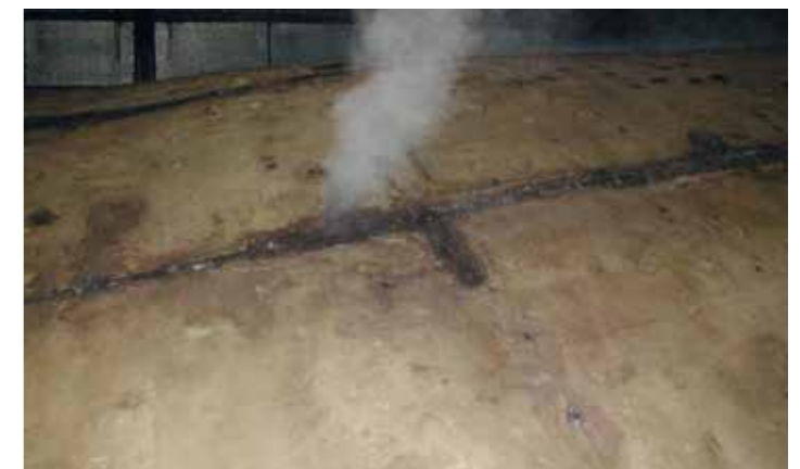
Process air escaping through a hole in the membrane.
