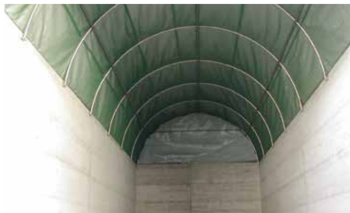
Variant 3: Box system with integrated membrane cover
