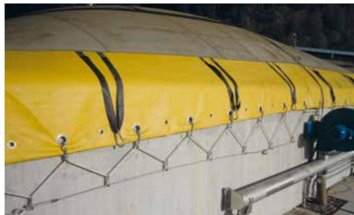
Variant 2: Drive-in silo with fixed membrane
